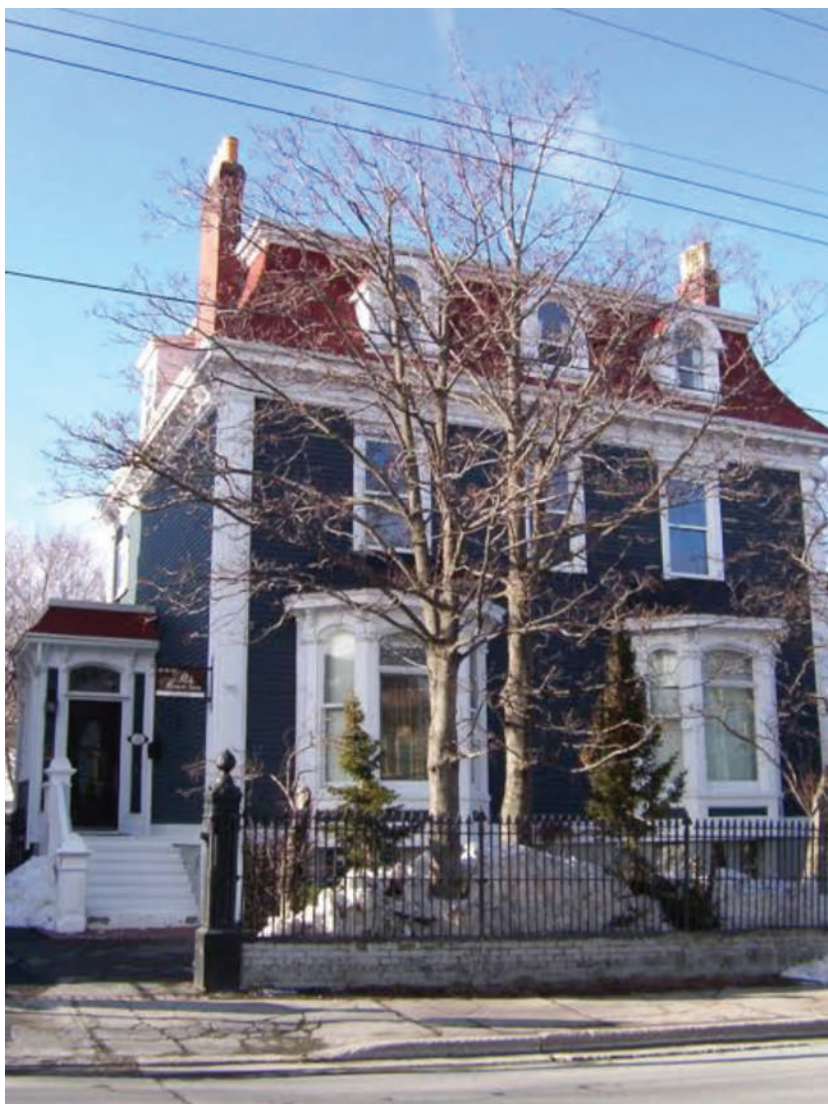
Exterior photograph of 112 Military Road – completed project.
