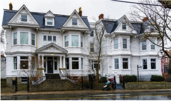
Ryan Mansion – Merchant's House – Bannerman Park Suites. Heritage restoration and adaptive reuse project incorporating a Five-Star Inn and eight luxury condominium suites.
